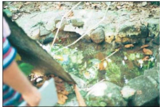
**Plate 1** (left) PVC drains from stream with rocks holding pipe in dug-out bed and forming a small check dam
